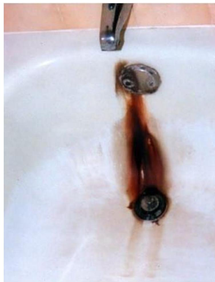
**Figure 1.** Iron and manganese staining
