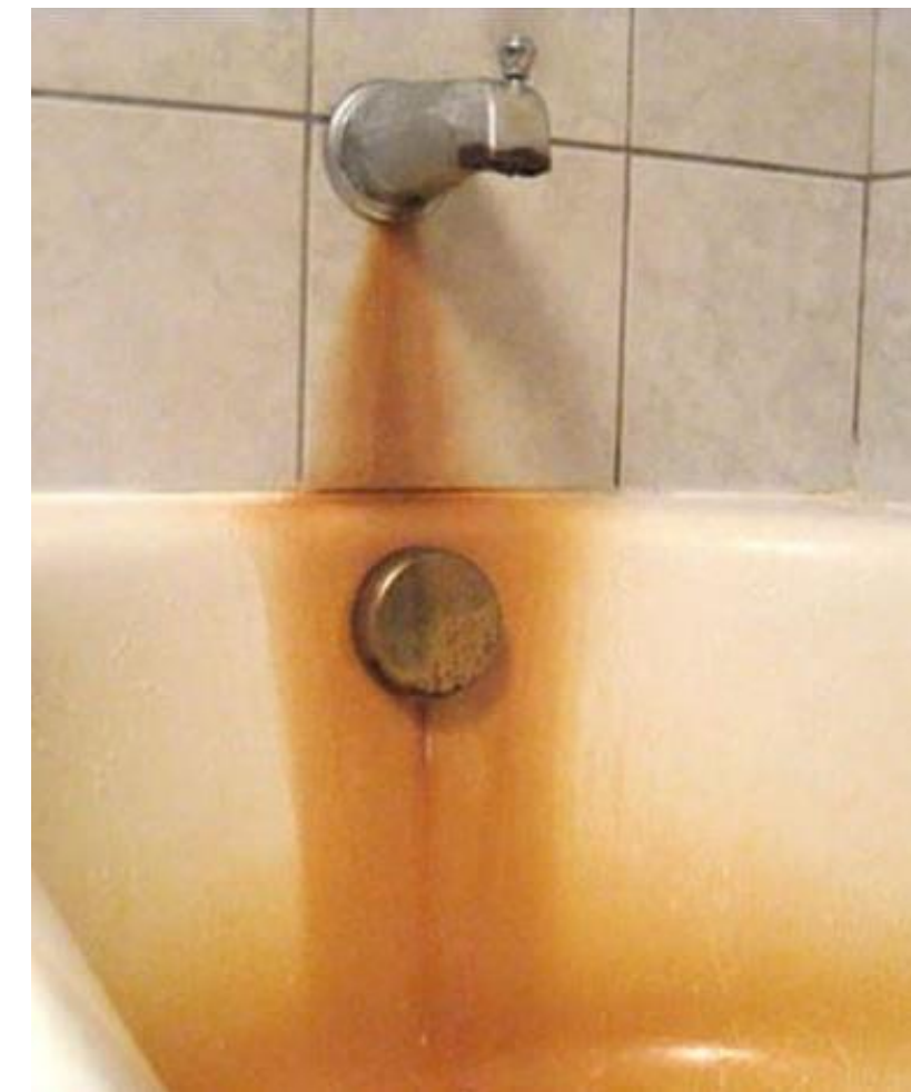
Figure 2. Iron staining
