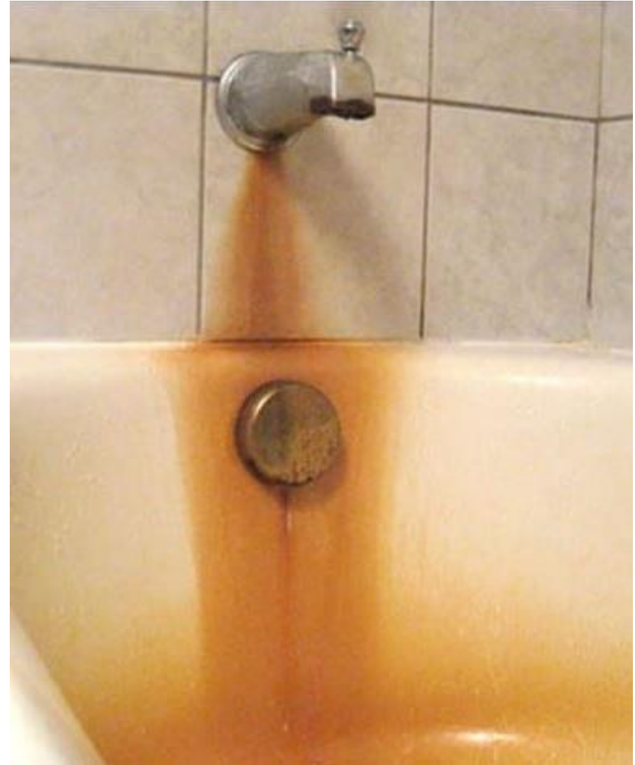
Figure 1. Iron staining
